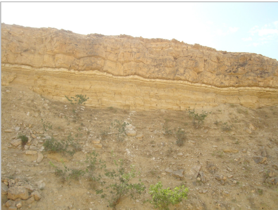
Figure 4. View of the Upper Cretaceous-Paleogene limestone outcrops on the NE limb of the anticline
