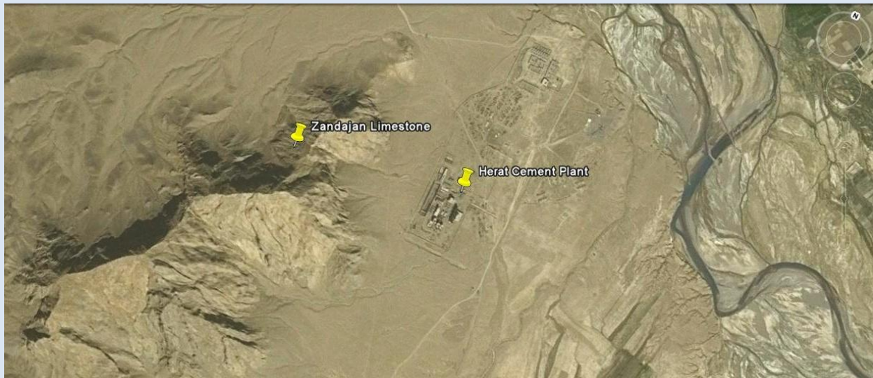
Figure 2: View of unfinished cement plant immediately across from the limestone-marl outcrops
